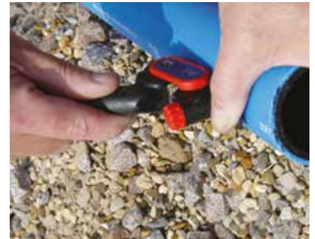
With light pumping movements, move the tool to the mark.
