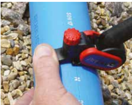
Rotate the tool by holding firmly with your thumb and remove the outer layer of the pipe.
