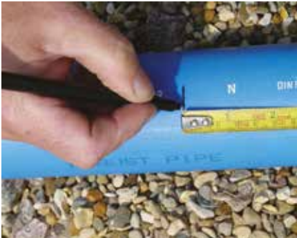
Measure and mark the pipe.
