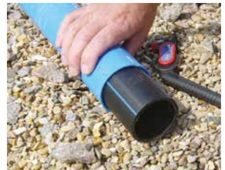
The inner layer is ready for smoothing and soldering (welding).
